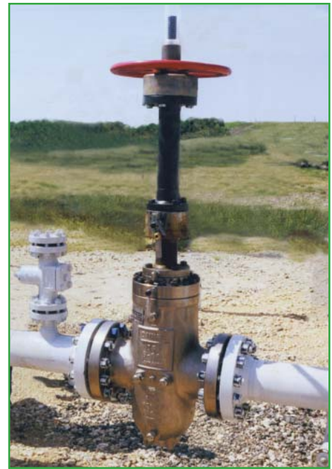
M&J EG Gate Valve with an emission-proof secondary stem seal design.
